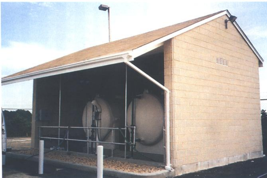
New liquid sodium hypochlorite (chlorine) bulk storage facility in Westhampton Beach.
