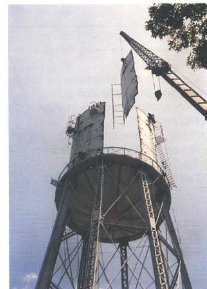
Dismantling old and obsolete water tank on Waterworks Road in Patchogue.
