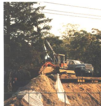
Portable drilling rig used to install replacement well at Washington Street Wellfield in the Village of Northport.
