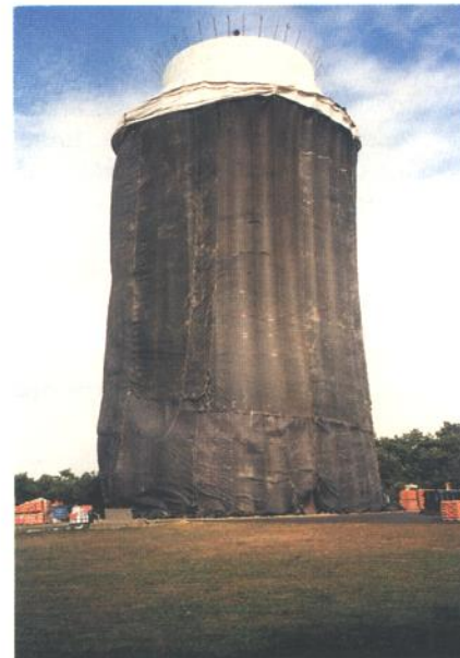
Sanding of Station Road Water Tank in Bellport (Containment structure totally encloses tank to prevent dust particles from being emitted into atmosphere).
