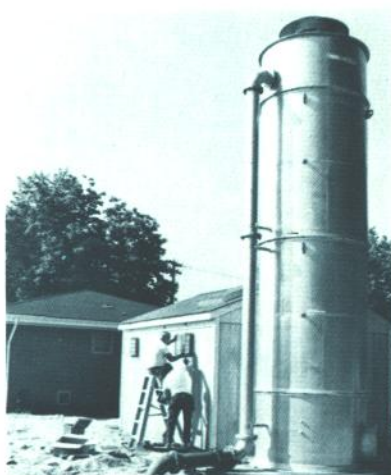
Finishing touches are applied to building housing electrical controls and well tank of new Air Stripping Plant designed to remove contaminants from water supply at the Bellrose Avenue Well Field site in Northport.
