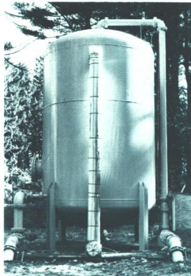
In service at the Long Springs Road Well Field site in Southampton is the first granular activated carbon filter to be utilized by the Authority in removing organic compounds from its water supply.
