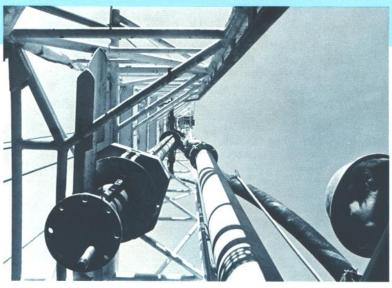
Drilling operations were underway on Well #1 at the Maple Avenue site in Medford.Well will be 360 feet deep,have a 20 inch by 12 inch diameter and be capable of pumping 1,300 gallons per minute. Total cost of the new well will be \$122,750.
