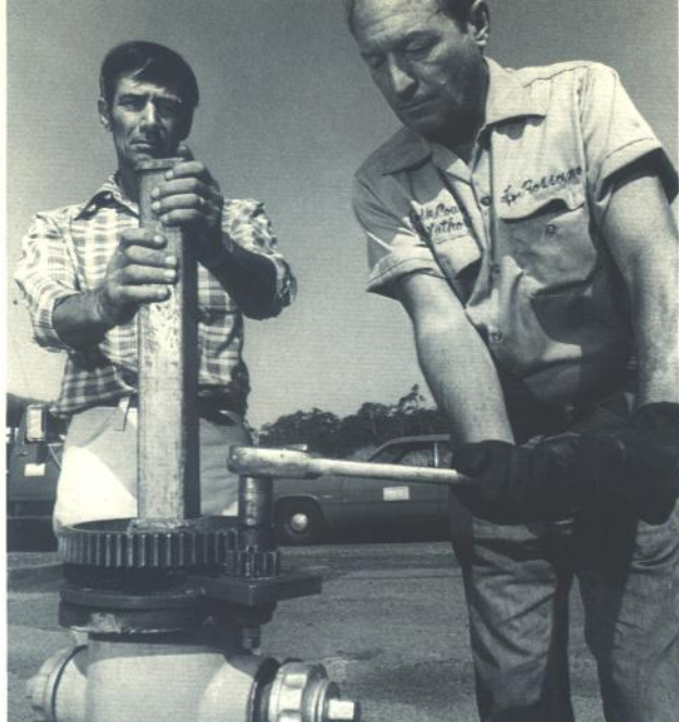
TESTING Port Hydrant Wrench are, right, Louis Rossano and Robert Radice, left, Authority employee who designed the new device. New device turns a two-man job into a one-man operation, cuts time spent freeing hydrant seat rings, and as part of the Authority's Safety Program, will help reduce job-related injuries to Authority personnel.
