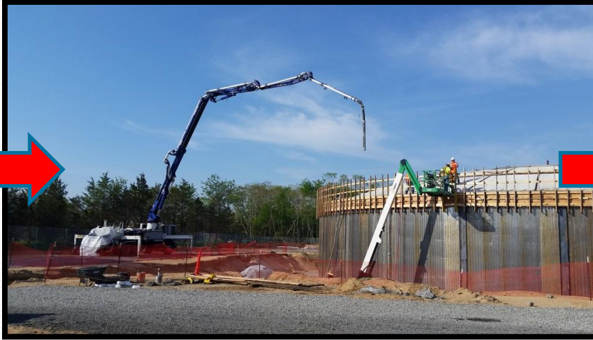
FORM AND POUR CONCRETE BETWEEN PANELS
