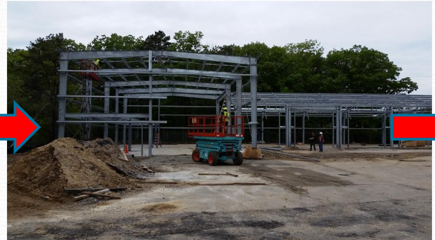
COMPLETE STEEL STRUCTURE
