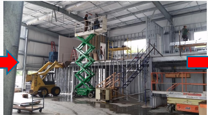
BEGIN FRAMING FINISHED OFFICE SPACE
