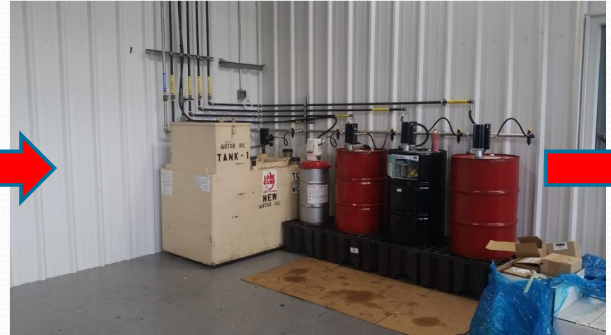
INSTALL BULK LUBRICATION FLUID SYSTEM
