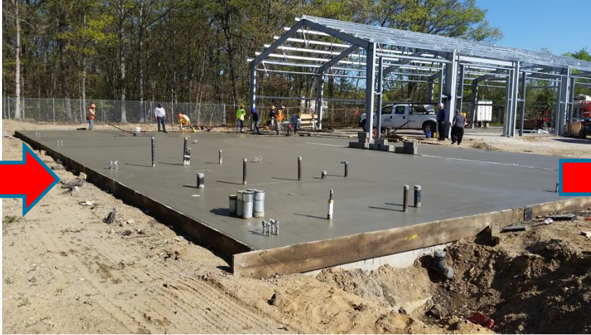
POUR THE SLAB FOUNDATION FOR BUILDING ADDITION
