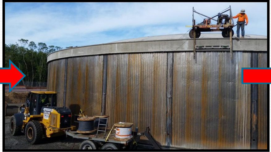
WIND TANK WITH STEEL CABLE
