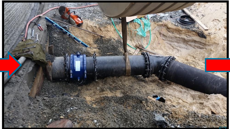
CONNECT TANK TO BOOSTER STATION
