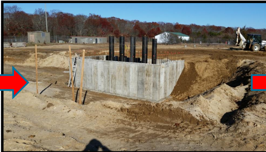
CONSTRUCT FULL DEPTH CONCRETE FOUNDATION & BACKFILL
