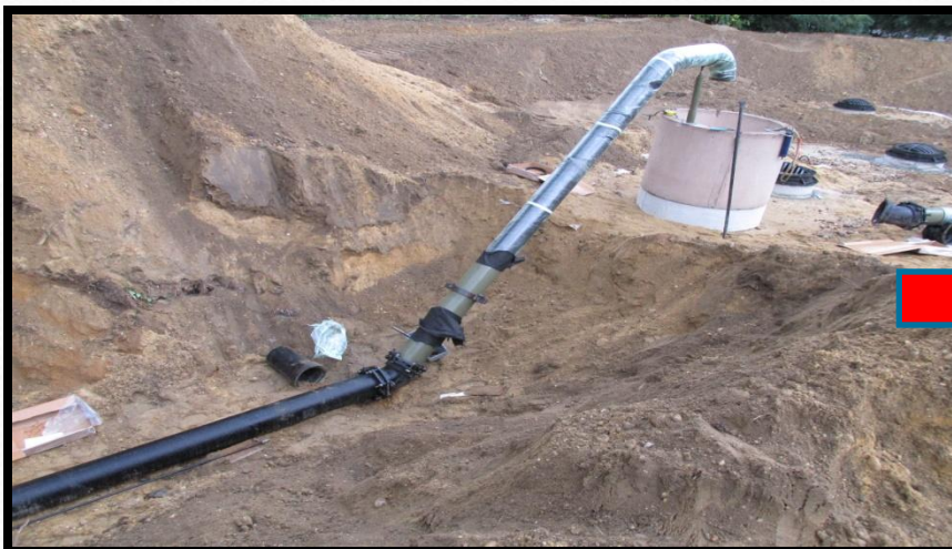
CONNECTING THE GOOSENECK
