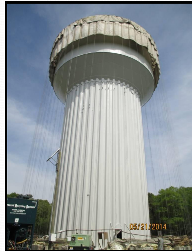
Sill's Road Tank Rehabilitation
