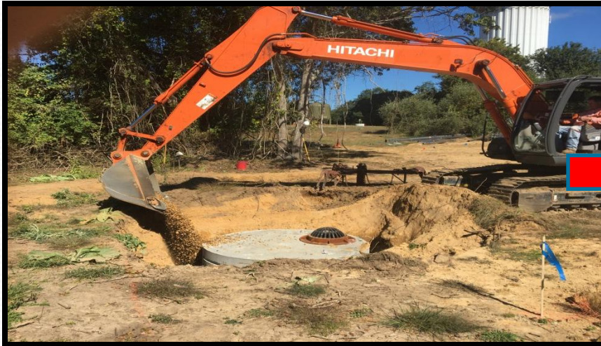
BACKFILLING
