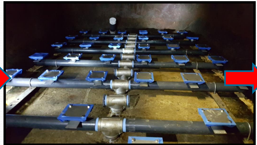
NEW UNDER-DRAIN INSTALL
