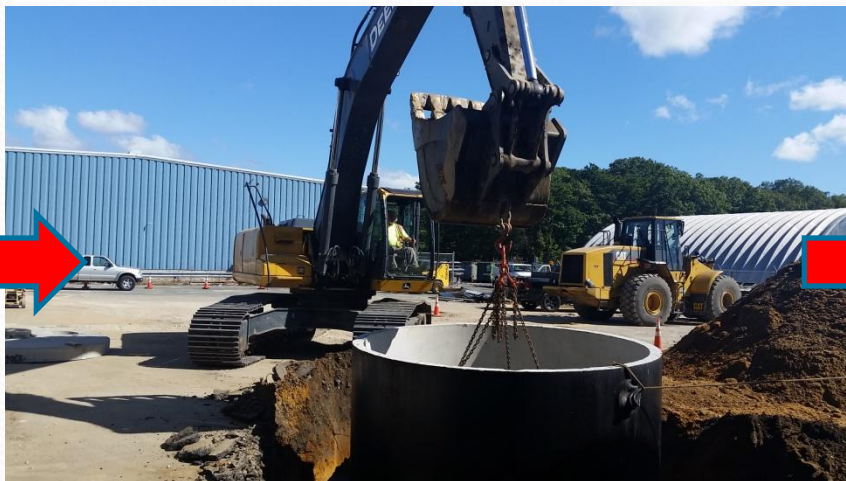
INSTALL THE SANITARY & GRAY WATER SYSTEMS
