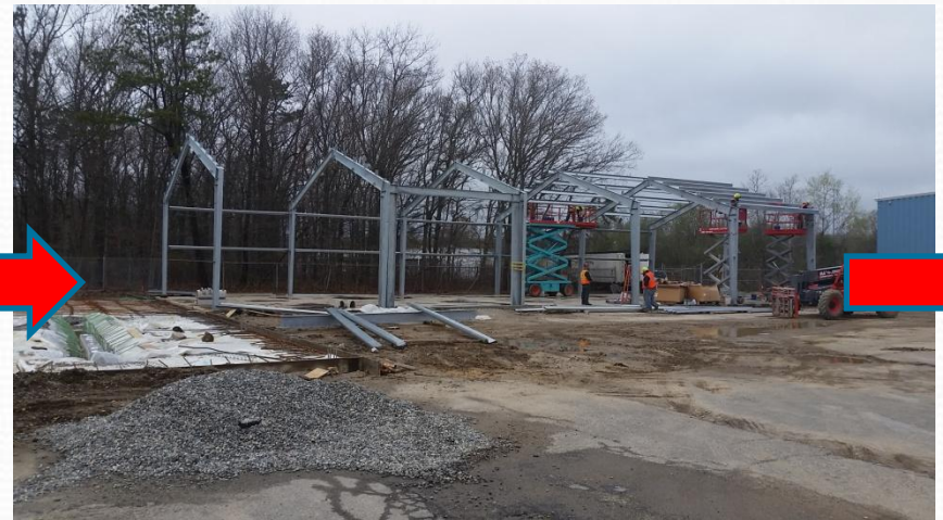
START ERECTING STEEL & PREPARING FOR ADDITION CONCRETE FOUNDATION POUR
