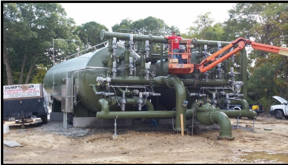
Easton Street I.R. System Construction
