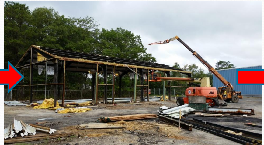
START ERECTING STEEL & PREPARING FOR ADDITION CONCRETE FOUNDATION POUR
