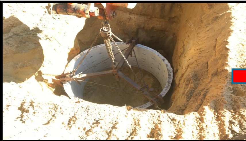
SETTING THE DRAIN POOLS
