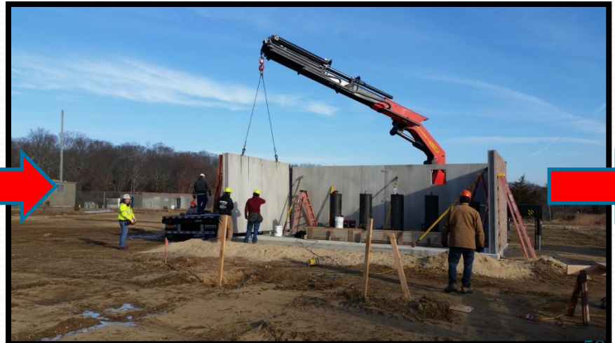
POUR THE CONCRETE SLAB FLOOR & SET THE BUILDING WALLS
