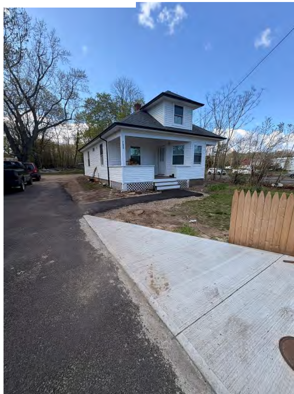
Photo 7: Residential building on parcel on corner of Cross River Drive and Main Road. Facing south.
