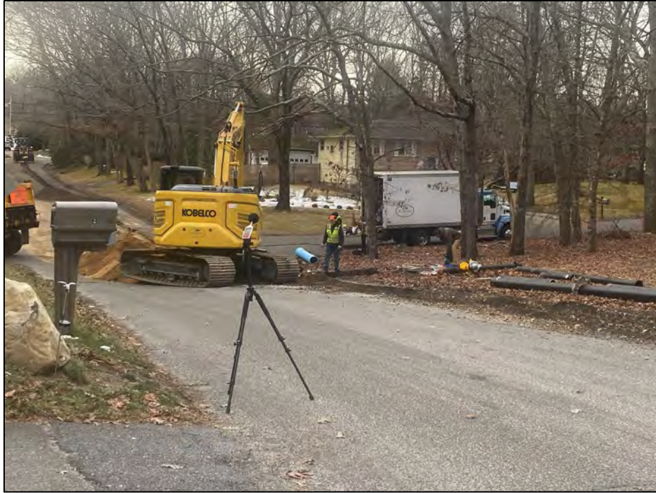
Photo 7: Active trenching occurring for a separate project, used to acquire noise data for the analysis of this report (1/23/26).
