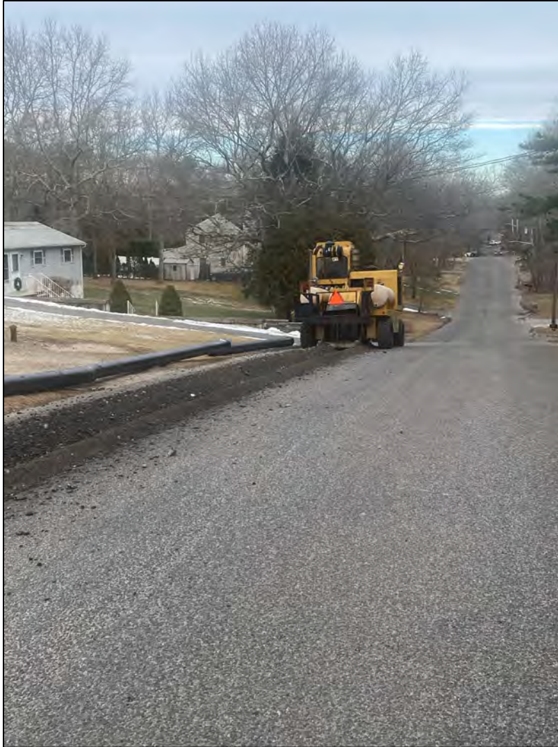
Photo 8: Active trenching occurring for a separate project, used to acquire noise data for the analysis of this report (1/23/26).
