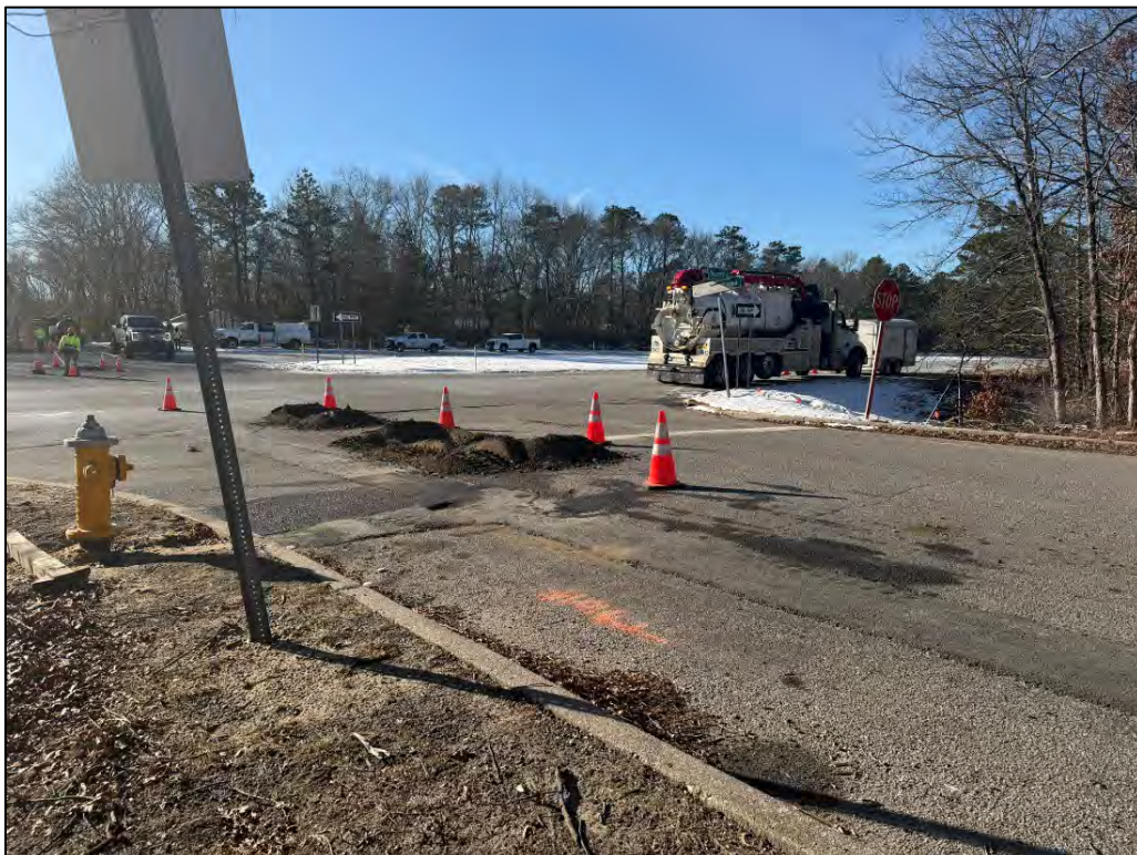
Photo 2: Showing the northern corner of Nugent Drive and Pinehurst Boulevard prior to directional drilling (1/21/26).
