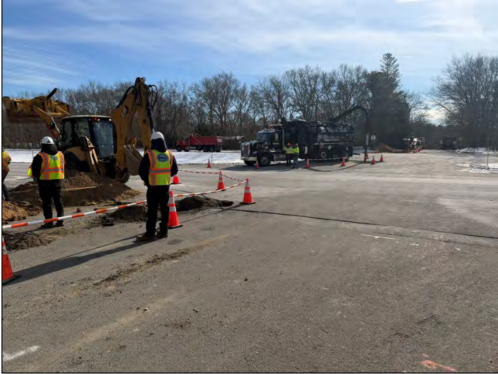
Photo 3: Showing active construction activities on the northern corner of Nugent Drive and Pinehurst Boulevard (1/21/26).
