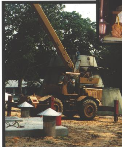
Contractors constructing tank in Huntington
