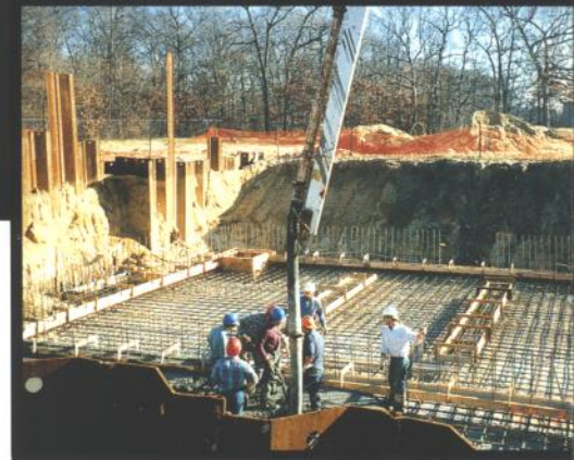
Constructing foundation of first iron removal plant
