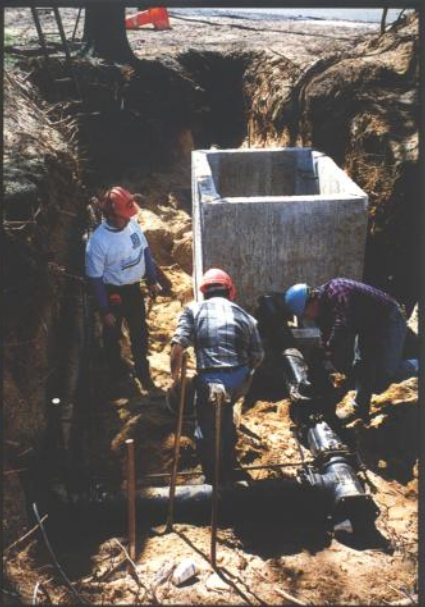
Contractors installing vault
