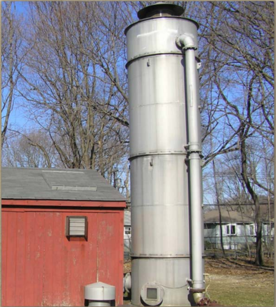
Air stripping operation located at Bellerose Avenue pump station in East Northport
