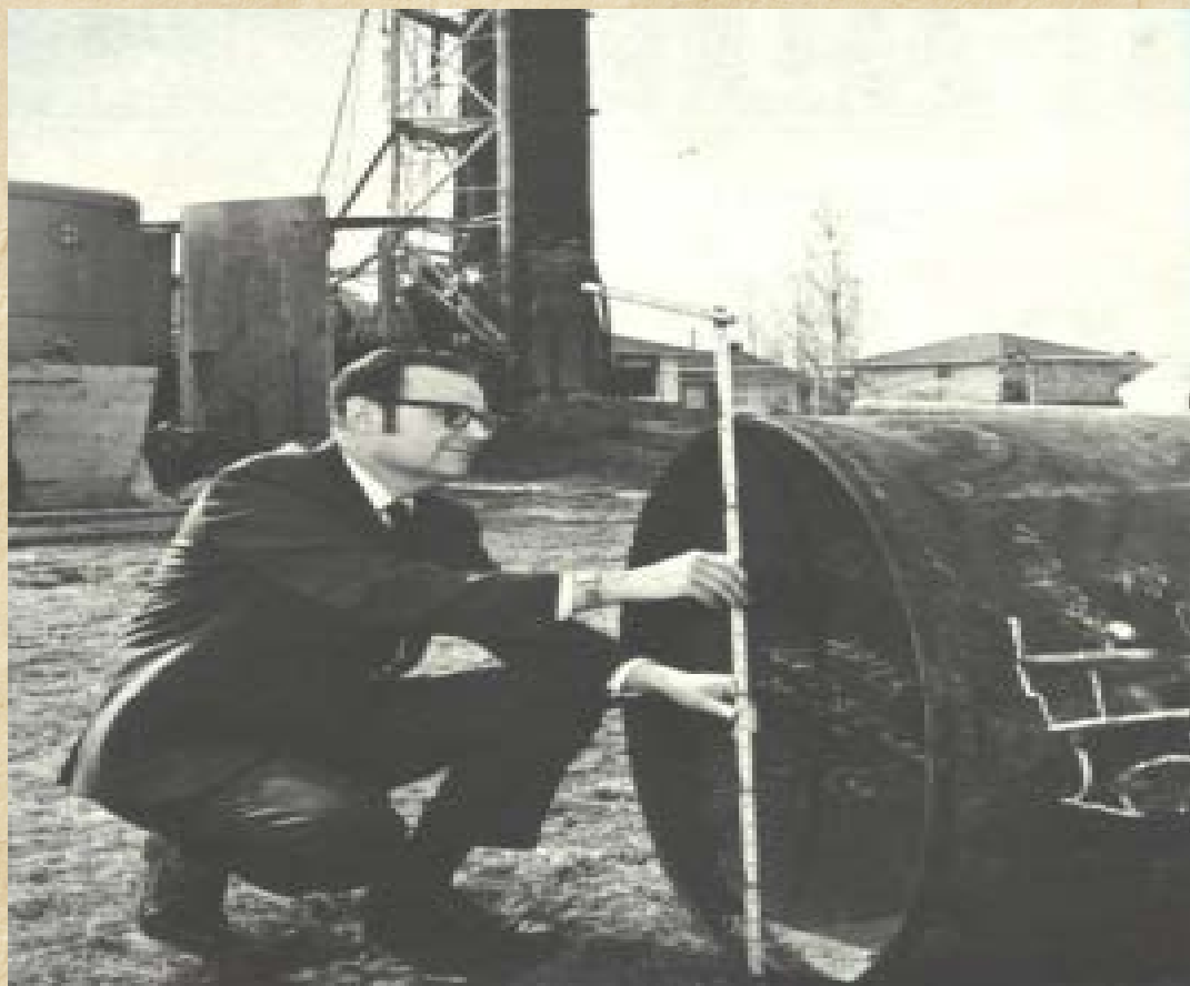
36-inch well casing is inspected by William J. Schickler, chief engineer of SCWA
